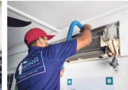
A technician with Wia Aircare Services, which has seen urgent requests for servicing increases by 40 per cent in the past three weeks, with most requiring an overhaul of the air-conditioning system. It also has to undertake more extensive work such as changing air-con pipes and condensers almost daily.
